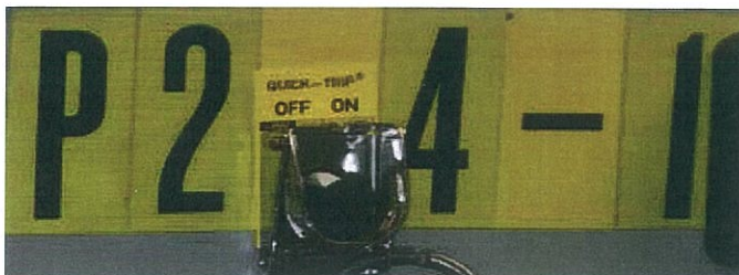
One of several Quick Trips located within the mill.
